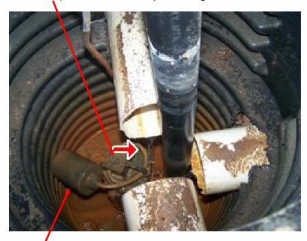
Float gets stuck between pump and sump walls
