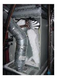
Investigation behind the service access panel in the furnace unit showed the inside AC coil was completely frozen. There was about 3-4" of ice on the coil, and no air flow or cooling was occurring.
