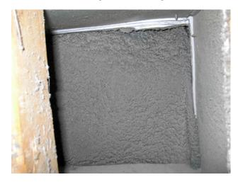
The cause? A dirty furnace filter... Replacing the filter is the simplest thing to do, but the most overlooked by homeowners. Replacement of the filter, and three days for the coil to melt = problem solved.
