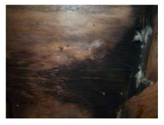
**Ventilation is the key...**the best solution to prevent this issue from occurring is proper attic ventilation. This could be roof top vents, soffit vents, gable vents, or a combination. An improper ventilated attic will allow moisture to condense on the interior sheathing, and be a recipe for mold growth. A proper attic inspection should include a review of insulation levels, structural aspects, proper ventilation, and the presence or lack of mold growth.
