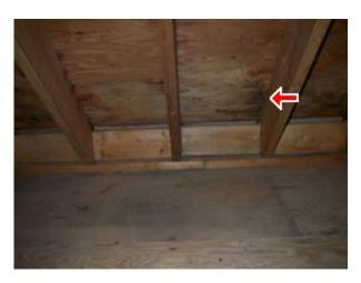
If mold growth occurs on the sheathing, and is allowed to continue, health issues can develop in the home, and eventually the roof sheathing can lose its structural strength.
