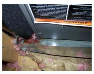
What wasn't clear was whether the leak had dripped down and damaged the ceiling below. No staining was evident visually. But, the Infra-Red camera was able to detect the presence of moisture in the drywall.
