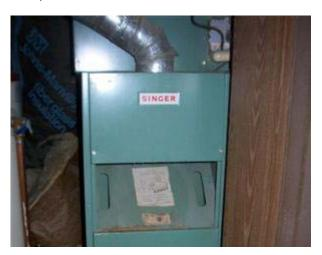
The right tool for this job is a combustion analyzer that can probe the flue, and measure the Carbon-Monoxide levels, Oxygen levels, and calculate operational Efficiency. Levels of Carbon-Monoxide measured in the flue should be less than 100 PPM (Parts-per-Million). This particular furnace was reading 1149 PPM of Carbon Monoxide in the exhaust flue!
