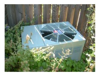
This unit might not operate very efficiently...if the growth around the outdoor unit is excessive, the air flow into the unit can be severely obstructed, and the unit will not function well. The compressor relies on adequate air flow, to help with the cooling process.
