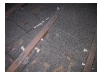
If this wiring is discovered in a home, usually in an attic or crawlspace, it will be recommended that this wiring be removed and upgraded by an electrician. This can be a considerable expense, but one that is necessary to prevent fires and prevent electric shock hazard.
