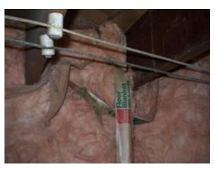
This wiring was used widely as the method for wiring a home. The hot and neutral wires are run as two separate wires, mounted on insulated posts (knobs), and run through insulated sleeves (tubes). This type of wiring was un-safe, as exposed connections could be contacted, causing possible electric shock to occur.
