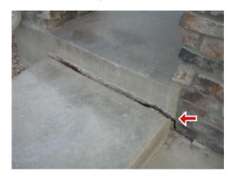
While some cracking is to be expected in our climate, this amount of settlement and cracking of the concrete is excessive. While mud-jacking may be possible, it is likely a full replacement of this walk will be needed.
