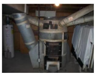
These heat systems relied on gravity to move heat through the home, and originally burned coal. The coal burner assembly is converted to a gas burner. Usually the ducts are wrapped with an "asbestos-like" material.
