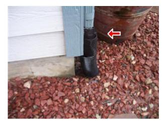
To prevent this from occurring, a simple cleaning of these buried lines with a hand-crank rooting device can push out any built up debris. This should be done at least once a year, in the spring or late fall.
