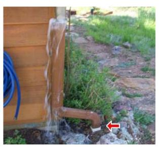
Keeping water away from the foundation is critical...if the downspout drain can't push water away from the home, there is a risk that foundation cracking or soil heaving can occur. This can go un-noticed for years, causing a significant and costly foundation issue.
