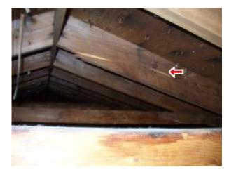
In this case, we had a split roof joist directly over top of the cracks. The homeowner had patched the cracks, but the cracks had returned, likely due to the snow loads and seasonal changes causing deflection in this area. The roof joist split was the cause, with this joist needing replaced, or a sister-joist added along side. When these types of cosmetic items are noted, further inspection is needed, to verify the cause.
