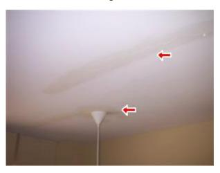
Attic's are inspected for not only insulation levels, leaks, and ventilation concerns, but when we see this type of ceiling cracking, it is important to inspect the rafter and joist system.
