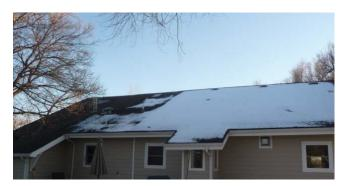
This was a north side roof, with the snow still present over half of the home, and the snow mostly melted on the other half. This is an indication that there is less insulation on the melted half, as the heat from the home is escaping easier, and melting off the snow quicker. This condition can lead to ice-damming and other issues on the roof, not to mention the loss of heat and comfort issues on this part of the house.
