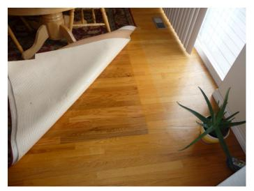
Wood flooring will lighten over time, as exposed to the sun. When rugs are down, the flooring under the rug stays at its original color. If the rug is removed, the flooring in this area will slowly lighten up, but it can take a year or more for this transition to occur. The alternative is to sand and refinish the flooring.
