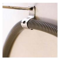
Imagine starting the dishwasher before you leave for work, and coming home to a nice puddle of water in your kitchen, potentially damaging adjacent flooring material and any surfaces below the dishwasher. A simple zip-tie or screwed on clamp will hold the drain line securely and prevent this issue from occurring.
