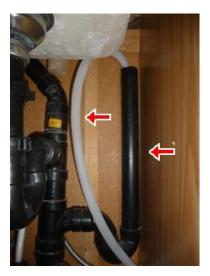
When the dishwasher runs, the pressure of the pump sending water through the drain line, can cause vibration and movement of this drain line. Over time, this drain line can come loose from the rigid drain pipe and could then start draining water in the cabinet area.
