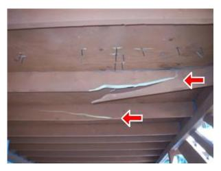
This deck has some serious structural issues present with the cracked joists, and safety issues with missing handrail guards.
