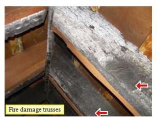
The roof trusses showed signs of extensive fire damage. While new framing members were added along side the burnt ones, there was a question of structural integrity.
