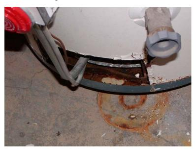
The most common mode of failure on gas-fired water heaters is for rusting to occur in the gas burner fire-pot area, where the vent pipe runs up through the unit, as shown below.
