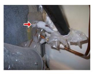
Once the coil is frozen, the air flow through the system becomes blocked, and the house will not cool down. The condensate drain system can overflow and leaks around the furnace can develop that can cause other expensive repairs. What's the most common cause of a frozen AC coil???
